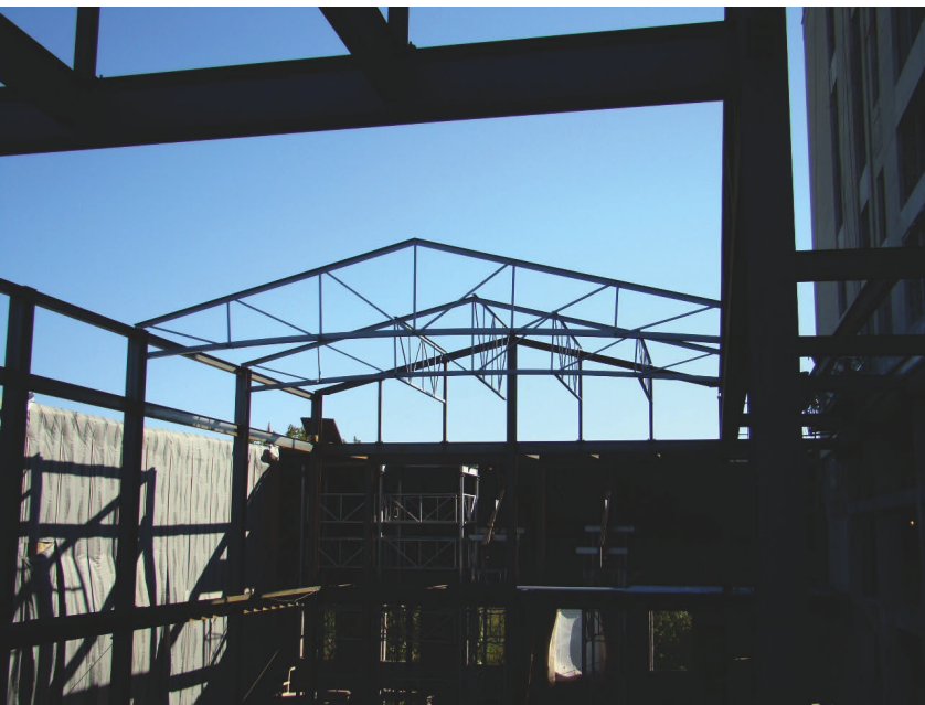
Skylight trusses at the east atrium.
