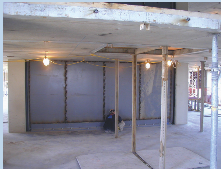
An SPSW in the library's stack tower.
